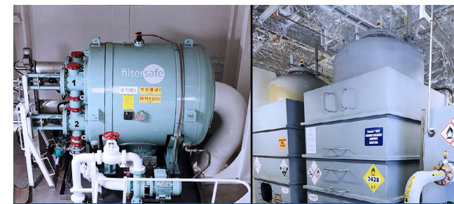
On-Board Ballast Water Treatment Installation
